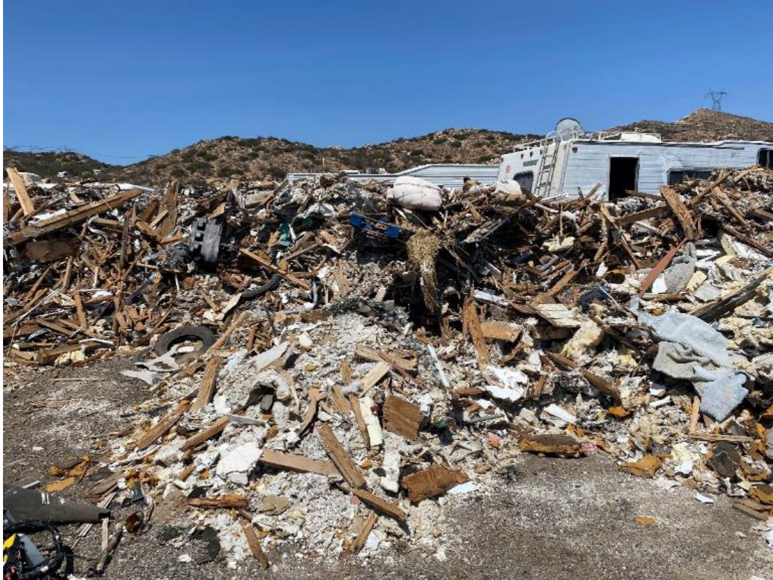
Potential ACM in construction debris, pile just southwest of previous pile
