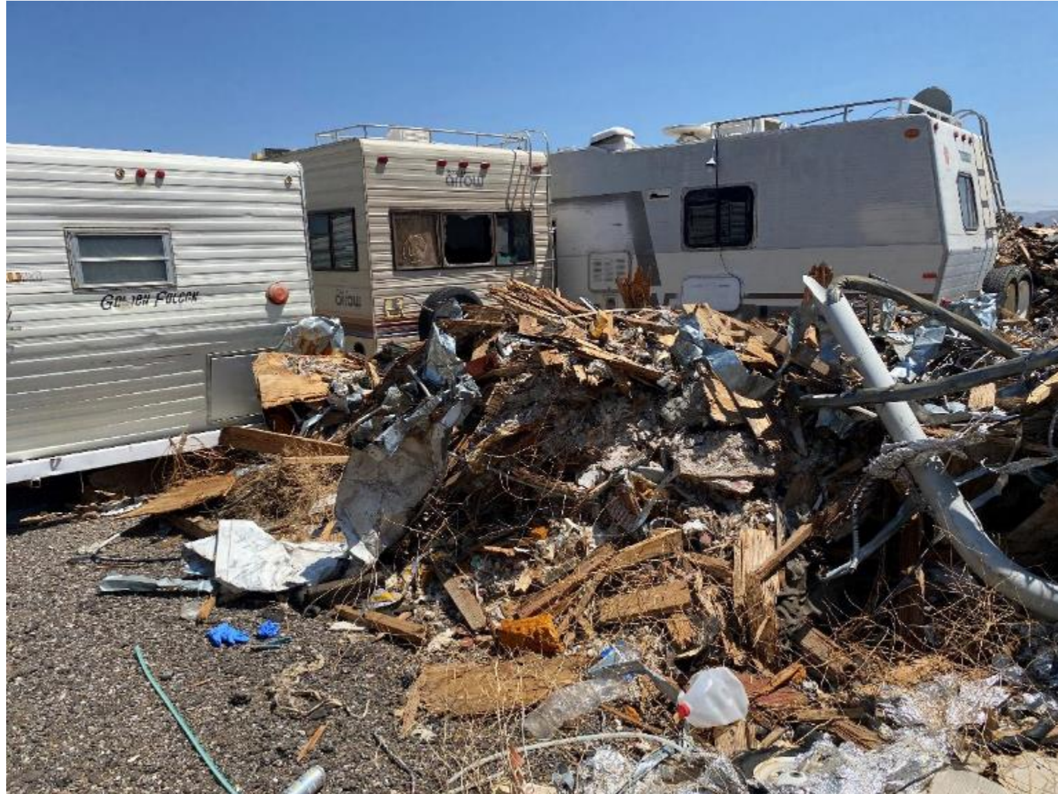
This pile on far northwest near RVs had some construction debris
