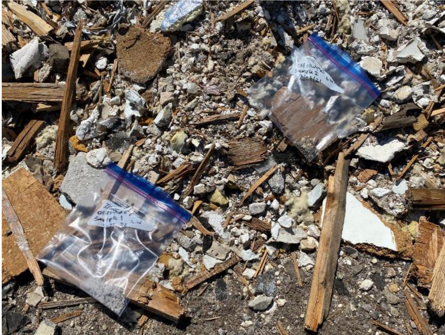
Potential ACM in construction debris
