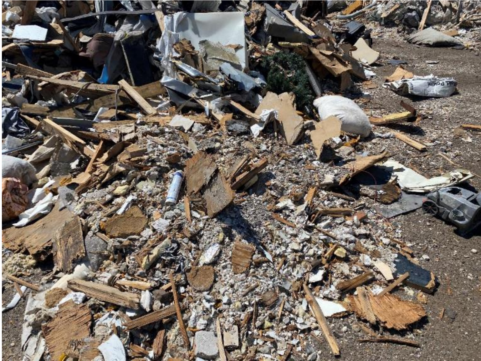
Potential ACM in construction debris
