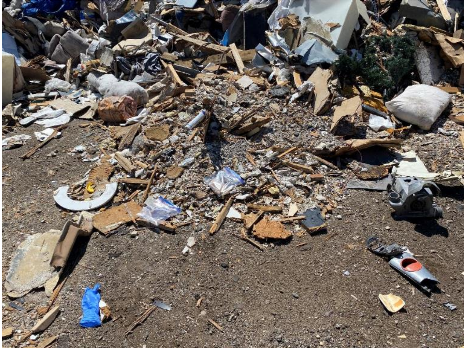
Potential ACM in construction debris, two samples taken, samples 1, 2
